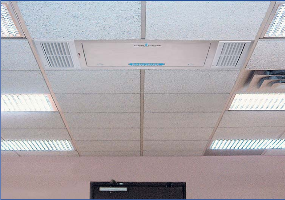
Figure 2 - The Sanitaire® Model RSCS280 (shown) is recommended for use in rooms with suspended "T-Bar" ceilings. Professional installation recommended.
